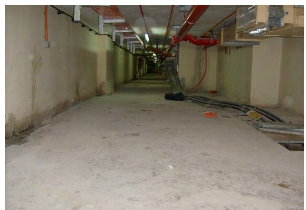
Both left and right photos shown the underplatform. The base slab of this underplatform was cast with Cementaid EVERDURE CALTITE and topped up with 100mm RC screed.
