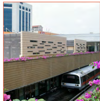
Precast wall blocks cast with Caltite installed at both sides of track
