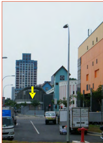
Photo to show that the new CCL MRT station indicated by yellow arrow is built close to the existing building.
