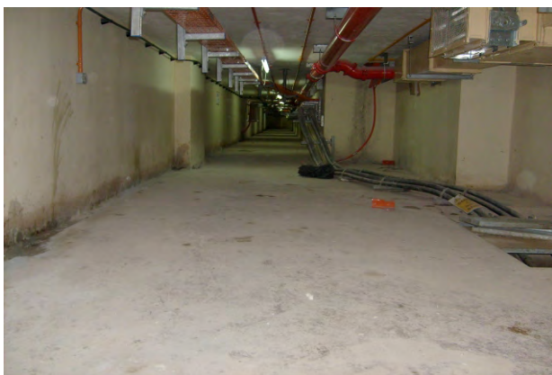
Both left and right photos shown the underplatform. The base slab of this underplatform was cast with Cementaid EVERDURE CALTITE and topped up with 100mm RC screed.
