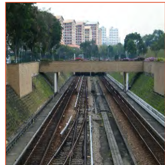
Precast wall blocks cast with Caltite installed at both sides of track
