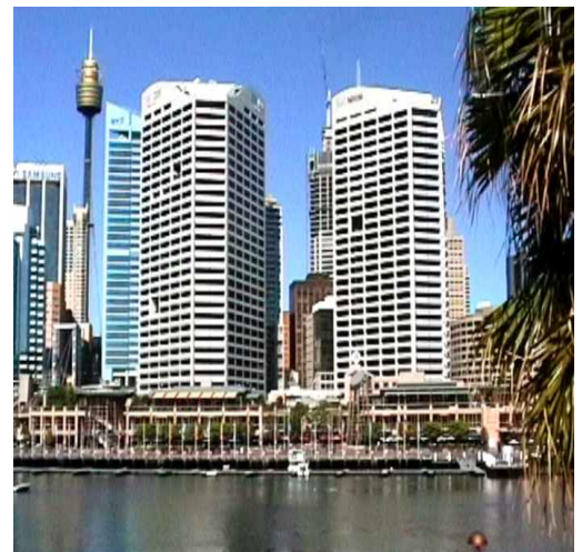
Darling Park, Sydney Membrane-Free “Caltite” concrete basements, up to 19m deep
